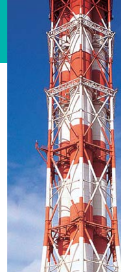
Chimney stack with heat-resistant protective coating
